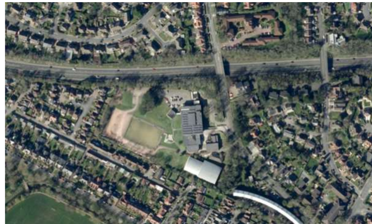
Aerial View of Existing Site
