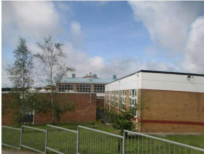
Figure 3. Typical External Façade of Existing Structure
