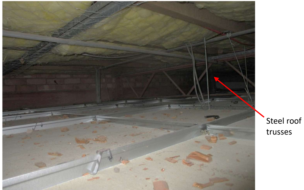
Figure 1. Roof Trusses Within Existing Building
