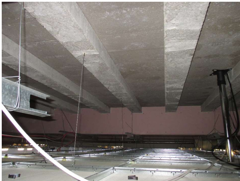
Figure 4. Precast Concrete Floors
