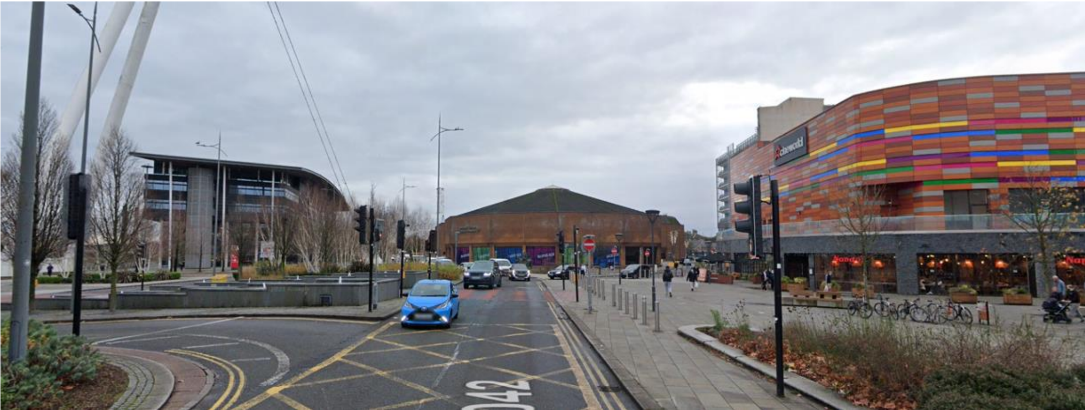
Figure 2 – View of the site from Usk Way looking south. The Friars Walk Shopping Centre can be seen to the right hand side and the University of South Wales to the left. The Kingsway Multi-Storey Car Park is in the background, partially hidden by the shopping centre. Source: Google Street View.
