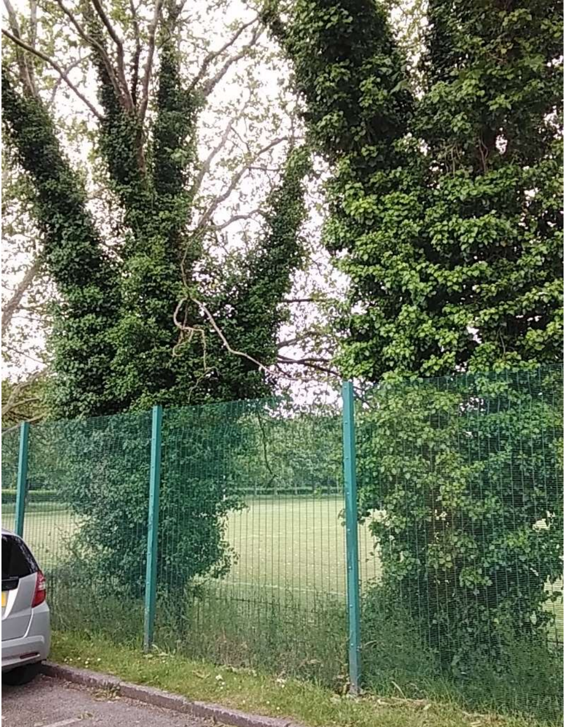
Photograph 1: G1- Ivy clad stems restrict inspection.
