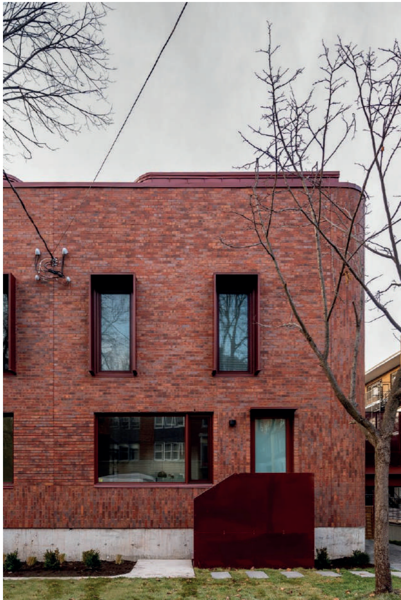
Window reveals and integrated shading surround Montreal Duplex Naturehumaine
