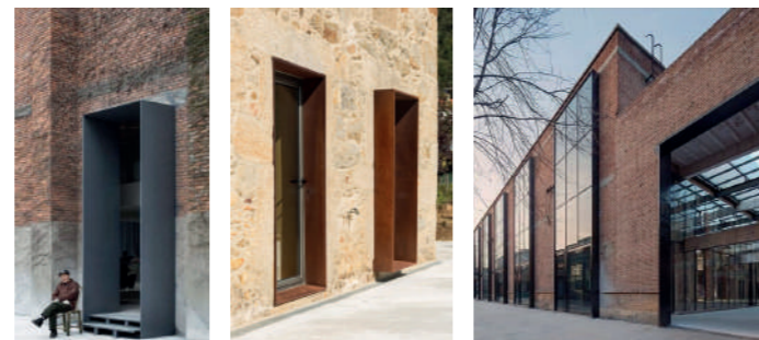
EXTENDED WINDOW FRAME REVEALS Reduces use of brick in reveals, keeping material palette simple.
