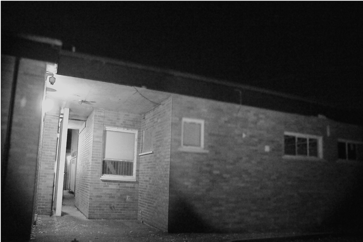
PLATE 2. Infrared lighting & Image during darkest time of survey on building K
