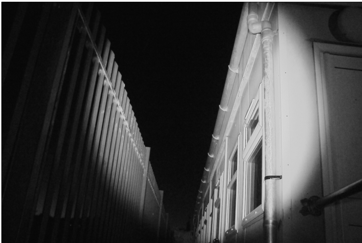
PLATE 22. Infrared lighting & Image during darkest time of survey on building D1
