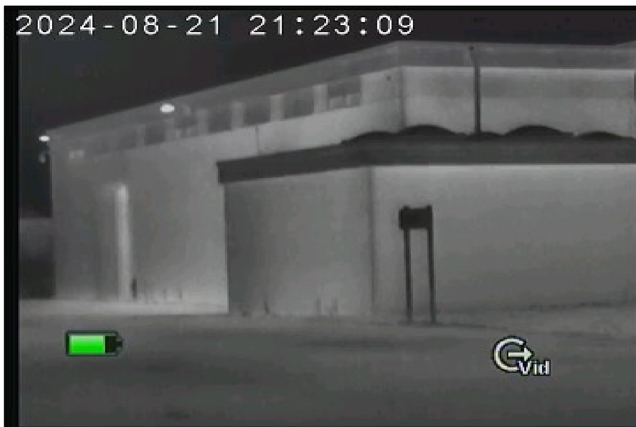
PLATE 20. Thermal image during darkest time of survey on building H
