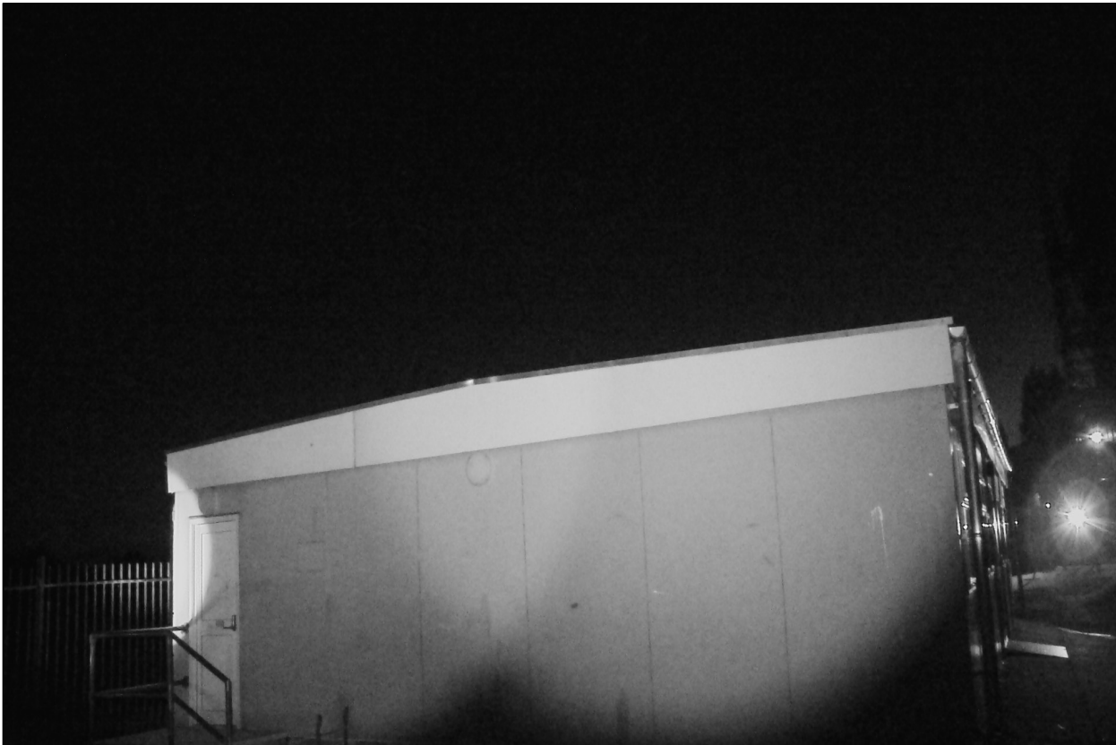
PLATE 12. Infrared lighting & Image during darkest time of survey on building D1
