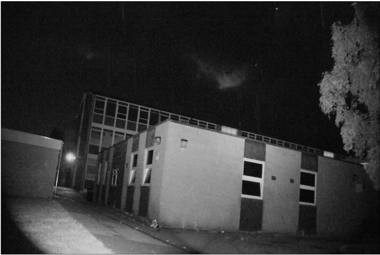
PLATE 8. Infrared lighting & Image during darkest time of survey on building G
