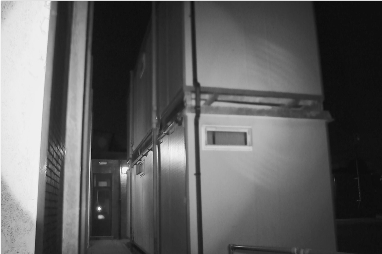
PLATE 3. Thermal image during darkest time of survey on building D3
