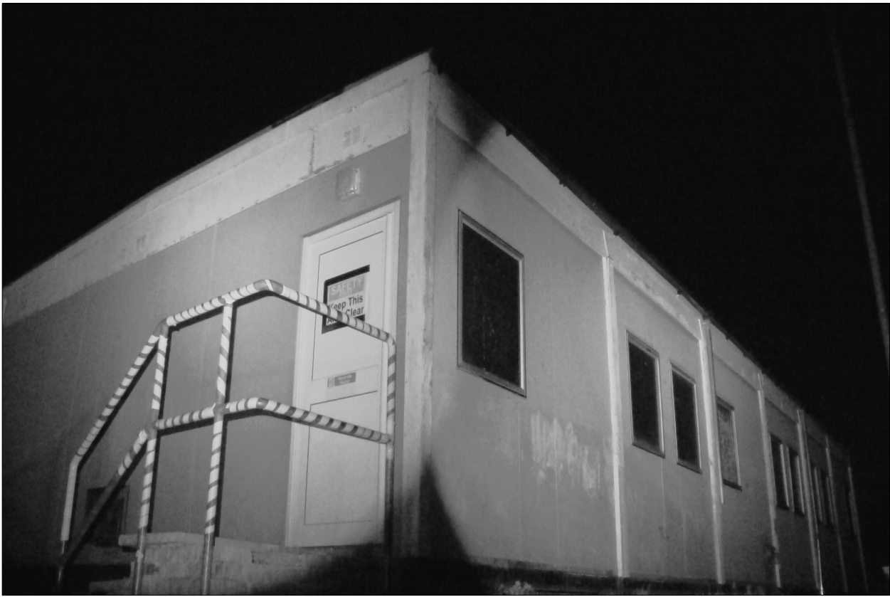
PLATE 24. Infrared lighting & Image during darkest time of survey on building D2
