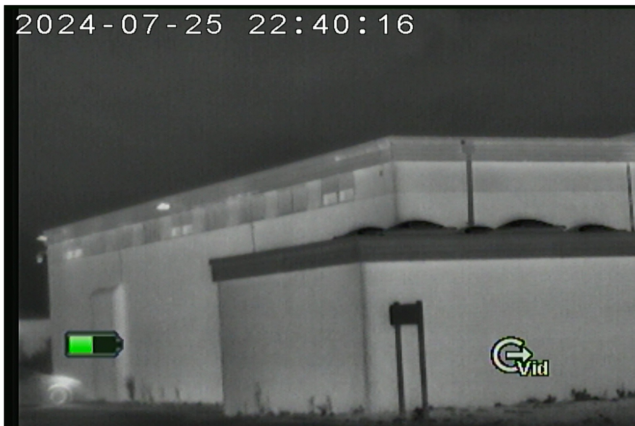
PLATE 7. Thermal image during darkest time of survey on building H
