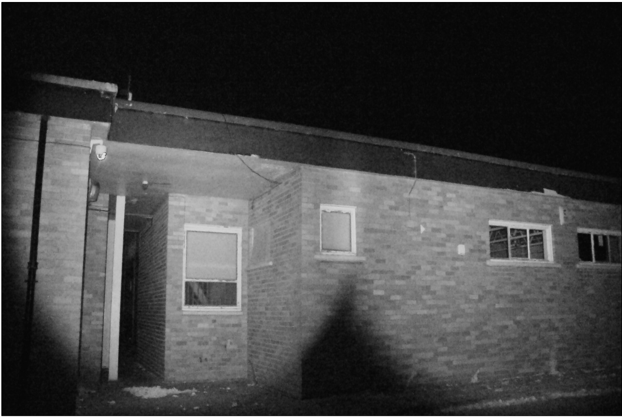
PLATE 18. Infrared lighting & Image during darkest time of survey on building K
