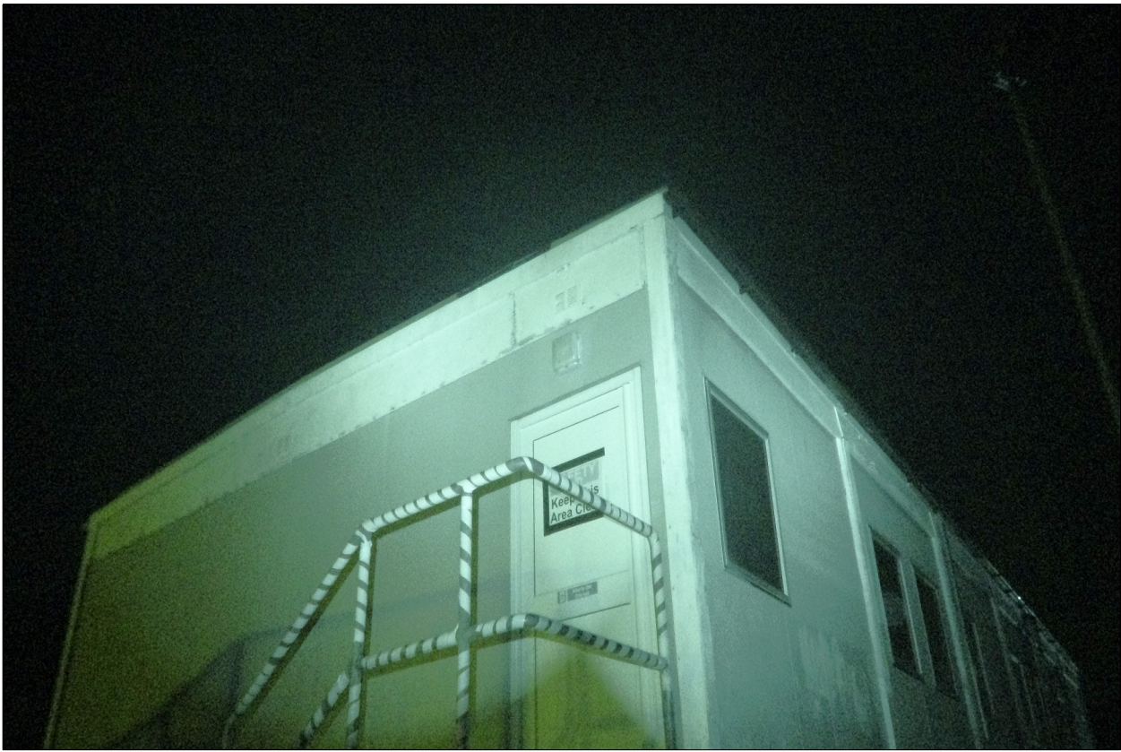
PLATE 15. Infrared lighting & Image during darkest time of survey on building D2
