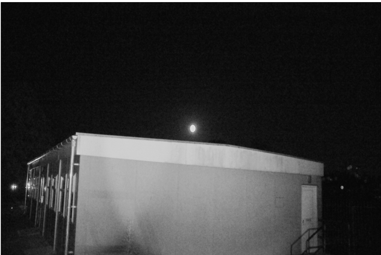
PLATE 14. Infrared lighting & Image during darkest time of survey on building D1
