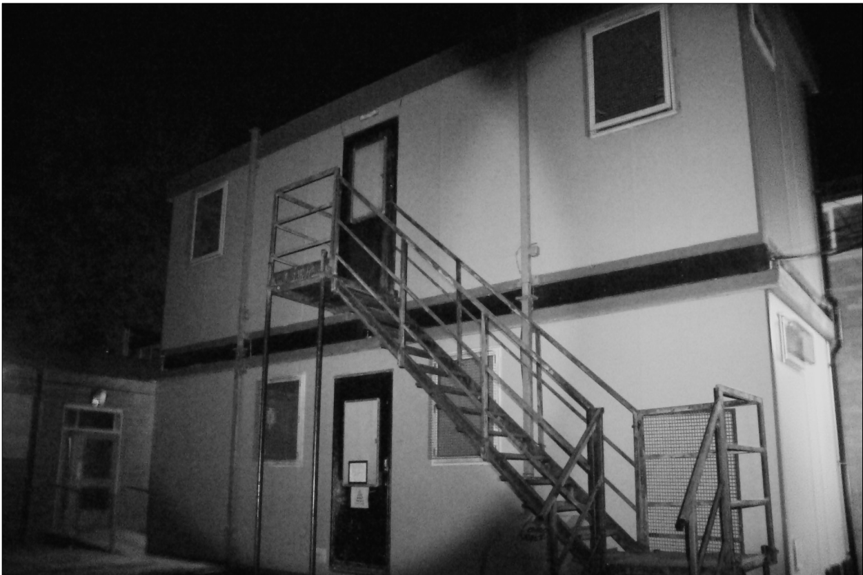
PLATE 4. Infrared lighting & Image during darkest time of survey on building D3
