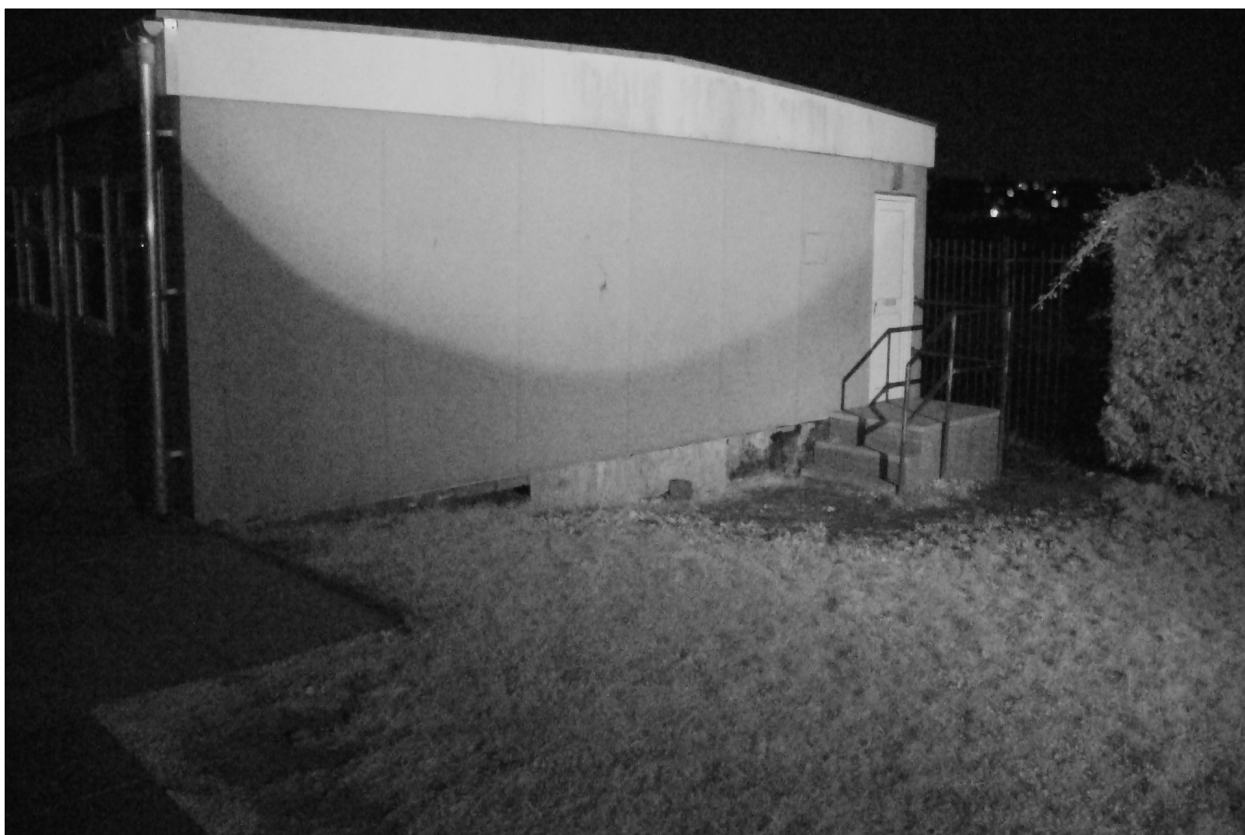
PLATE 23. Infrared lighting & Image during darkest time of survey on building D1
