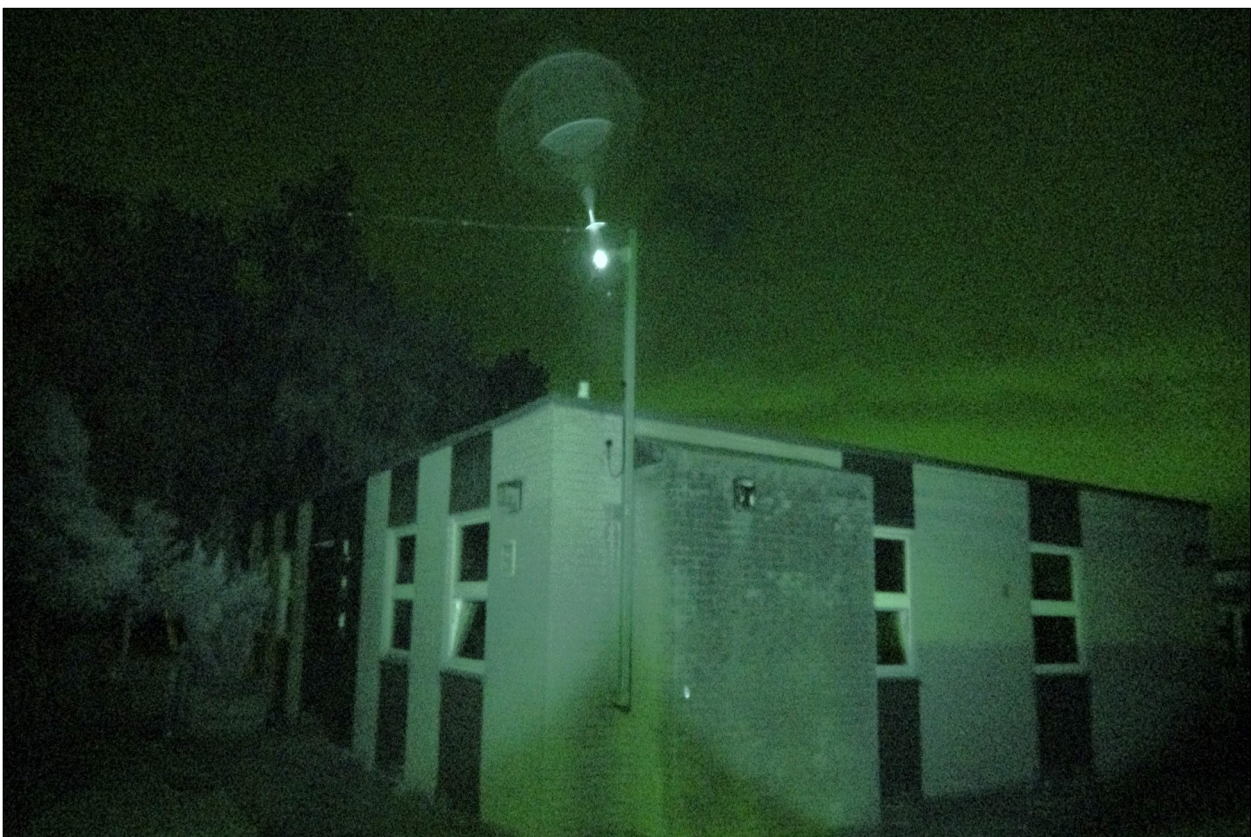
PLATE 11. Infrared lighting & Image during darkest time of survey on building G
