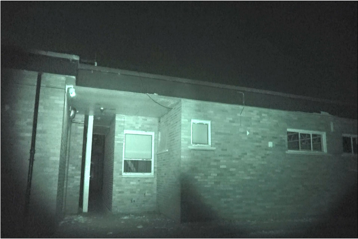
PLATE 26. Infrared lighting & Image during darkest time of survey on building K
