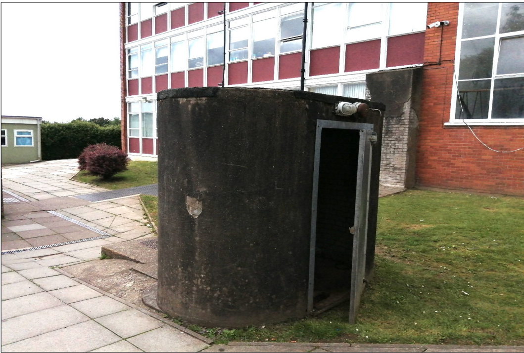
PLATE 14. A small rendered brick building (Target Note 10)
