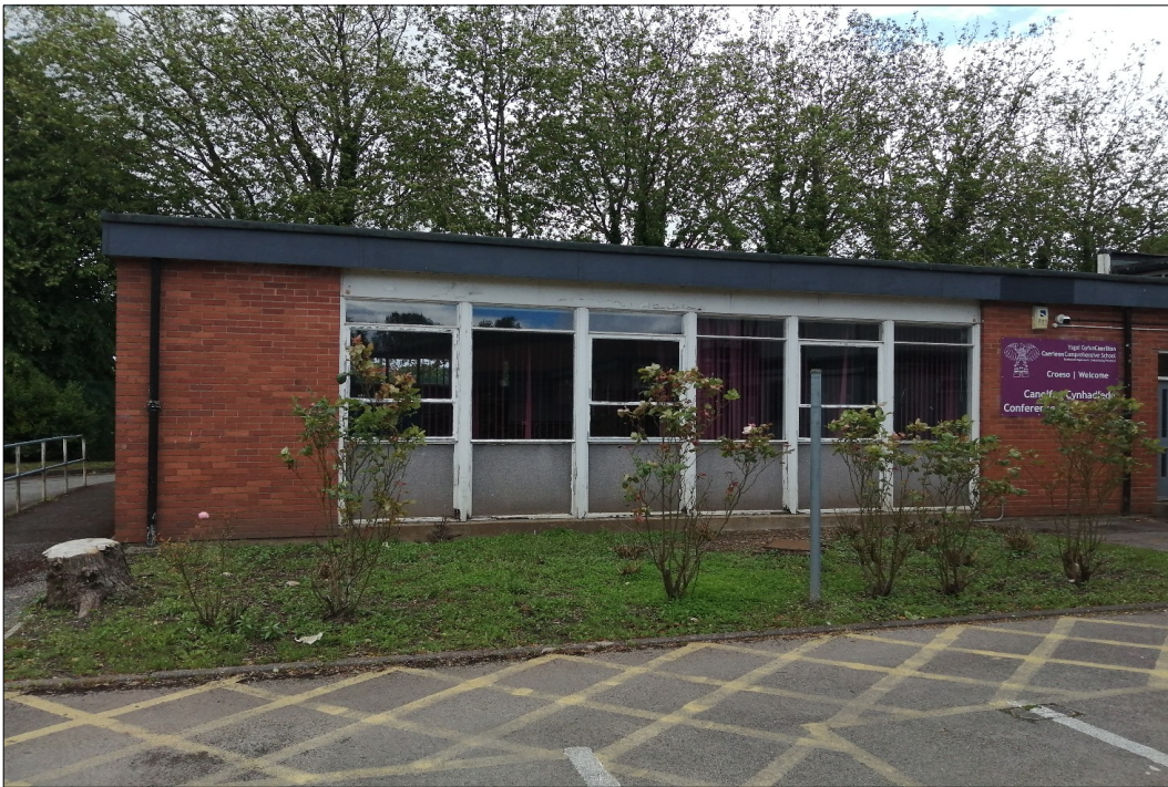
PLATE 4. Building K – Conference building (Target Note 2)
