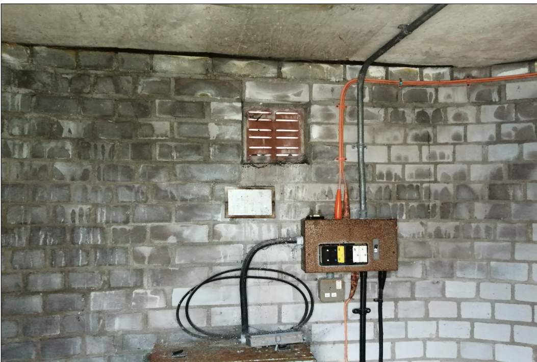
PLATE 15. A small rendered brick building (Target Note 10)
