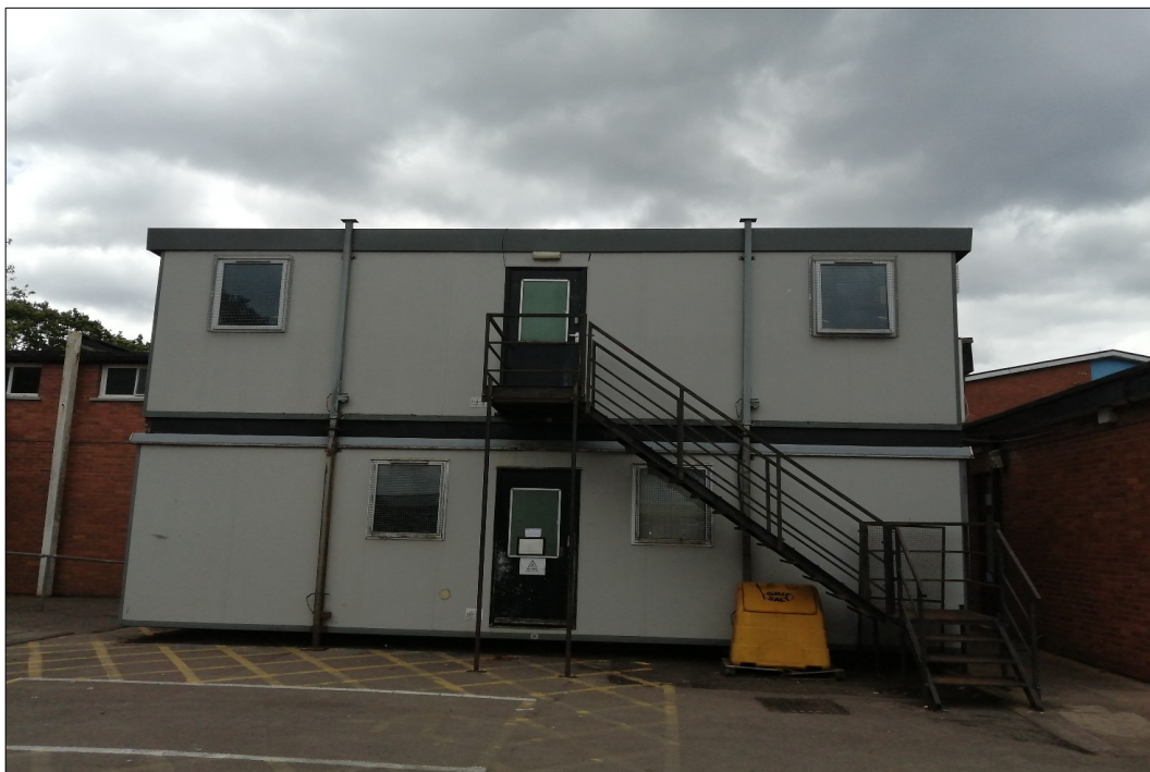
PLATE 1. Building D3 - Porta-cabins stacked on top of each other (Target Note 1)
