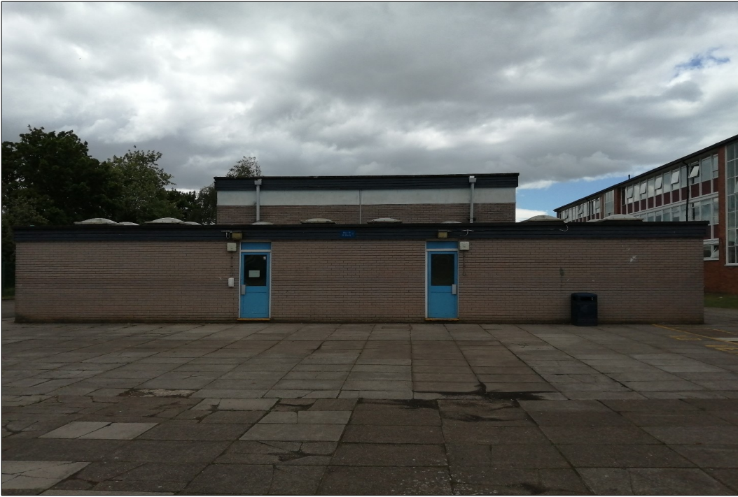
PLATE 10. Building H – Gym (Target Note 7)
