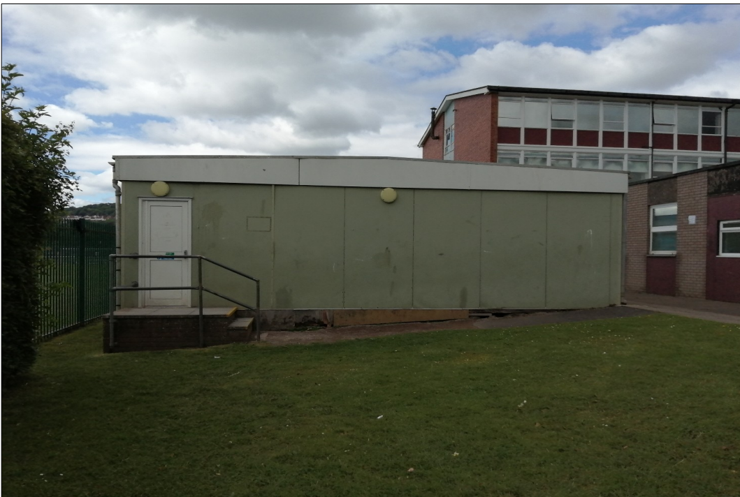
PLATE 17. Buildings D1 & D2 – Drama & learning hub porta-cabins (Target Note 18 & 19)
