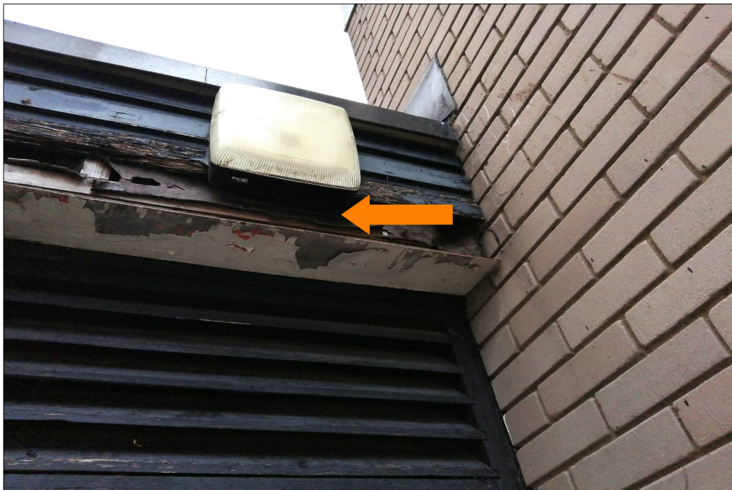
PLATE 13. Building H – Gym showing rotten soffit box (Target Note 12)
