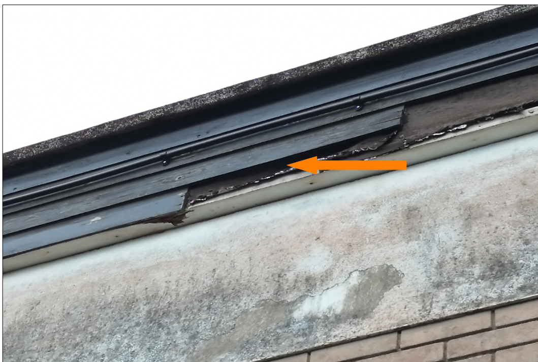
PLATE 13. Building H – Gym showing rotten soffit box (Target Note 12)
