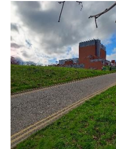
View 3. Northern site boundary from the north east.
